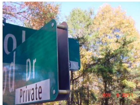
Figure III-8 Oversize Sign Showing Corner Attachment Detail
