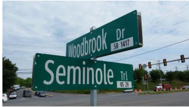
Figure III-6 Oversize (12'') Sign Showing Direct Mount Method
