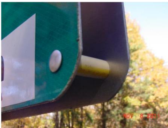
Figure III-7 Oversize Sign Showing 2'' Spacer (Gab) Detail
